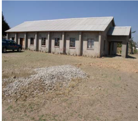
Church Building near Completion
